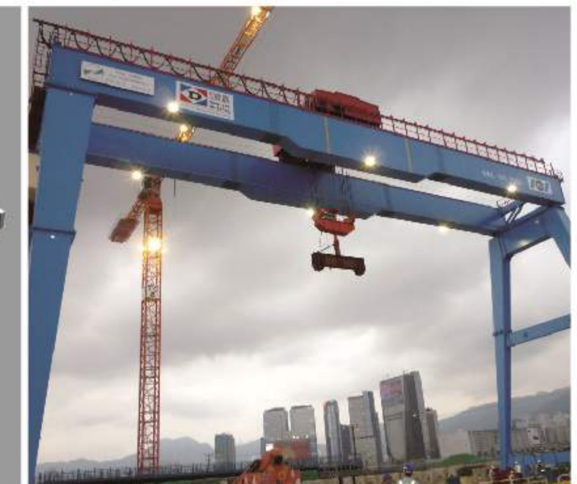
2011 Hong Kong Cruise Terminal 150 Tons Gantry Crane Project
