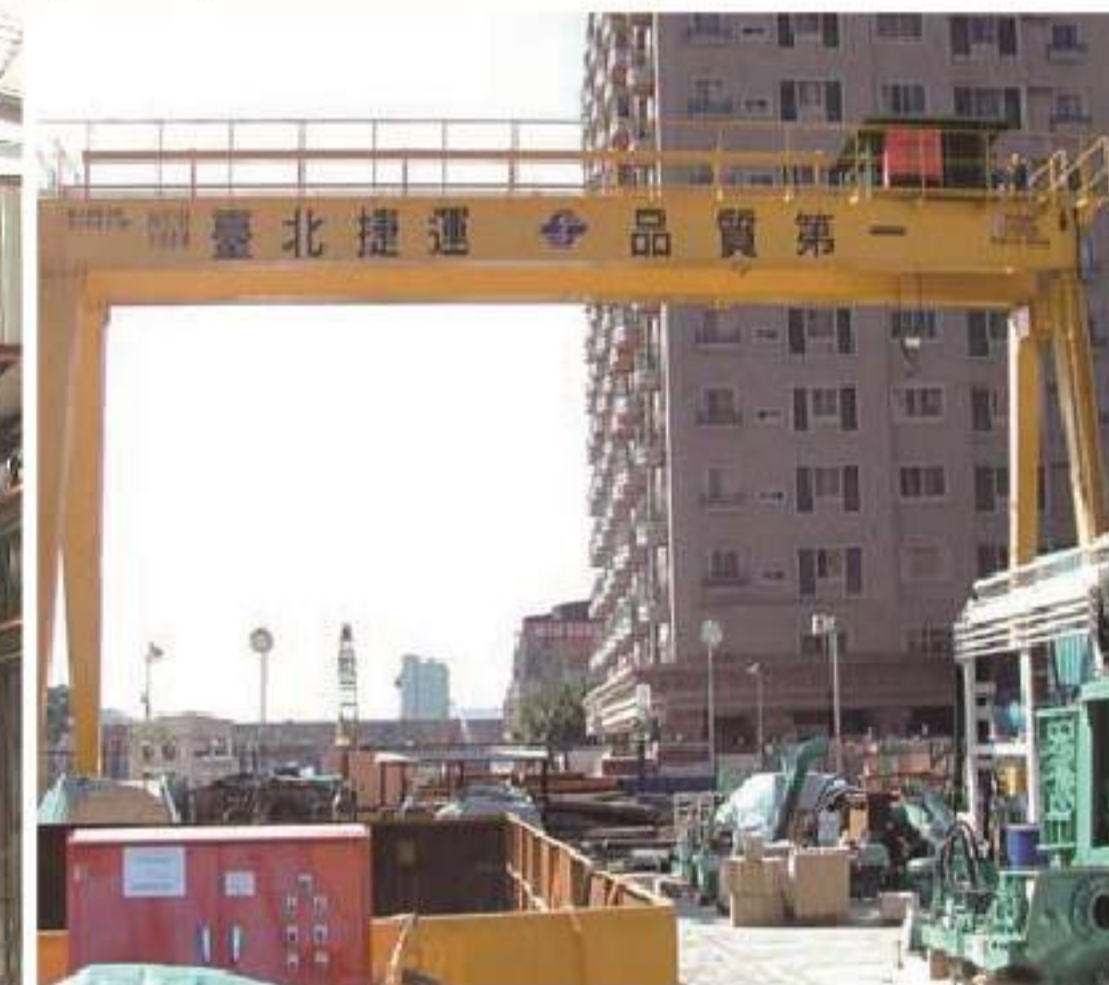
2005 Taipei MRT 10 tons crane
