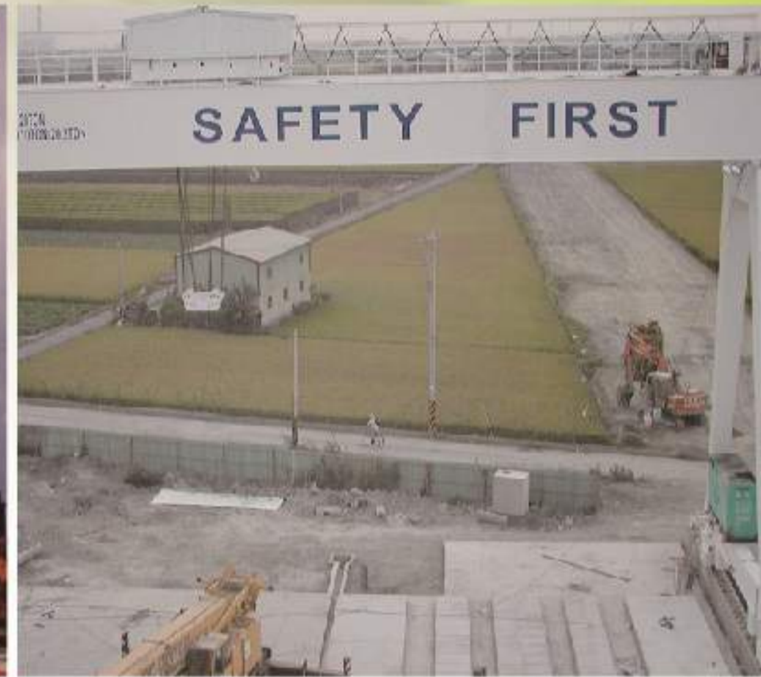
2001 Taiwan High Speed Rail 100 tons gantry crane
