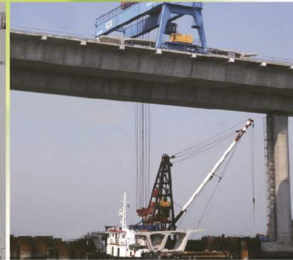
2004 VSL Hong Kong 150 tons gantry crane, lift height= 50M
