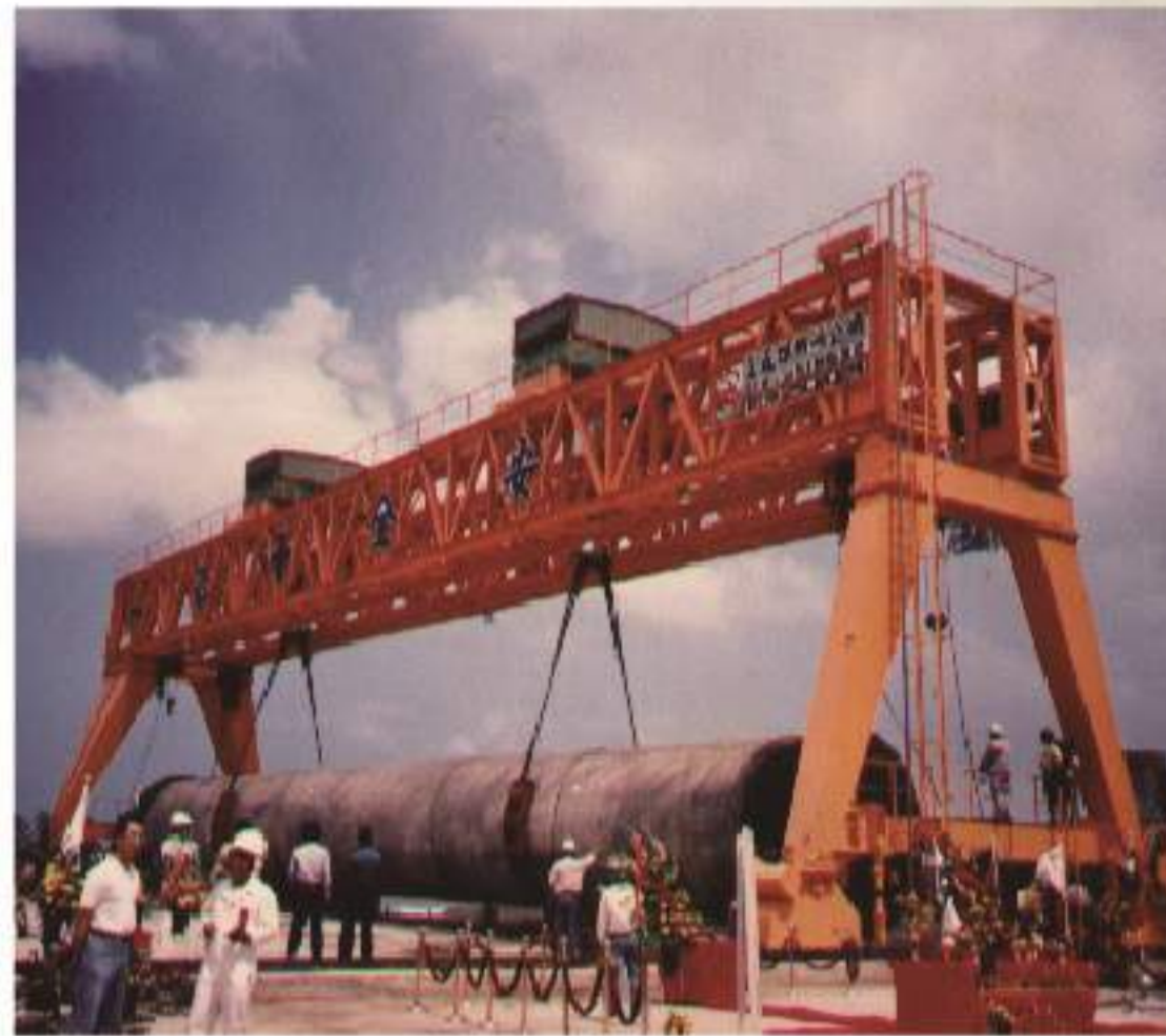
1988 Bali, Taipei 200 tons crane project
