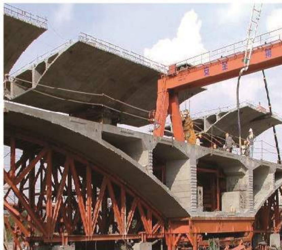
2000 Highway (Kuaiguan sections) Asia's largest bridge
