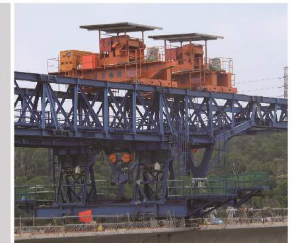
2011 Hwang Chang General Contractor Co., LTD. C911 Project 80 Tons Crane
